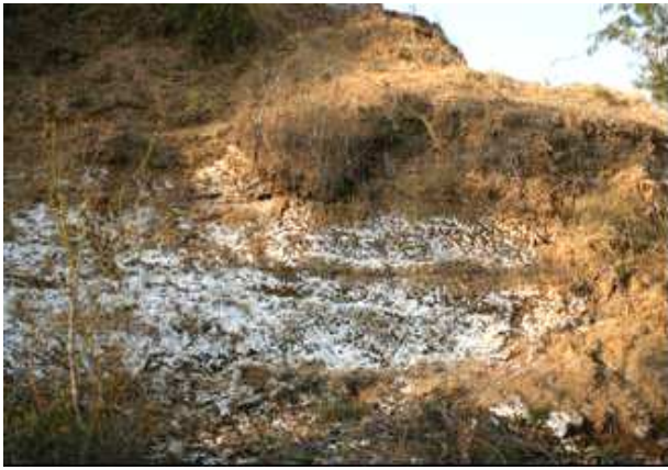
Fig. 6. The precipitation of alkaline salts in a place of groundwater seepage which was active in the wet season.
